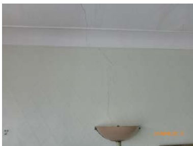
Cracks to the wall at the joint to the main building
