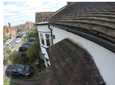
Cracked mortar to box gutter flashing Cement fillets to all edges and abutments are poor
