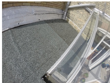
Rear shed roof is poorly felted and the flashing is poor
