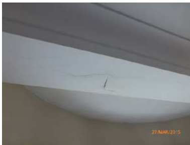
Water damage and staining to the drop down beam
