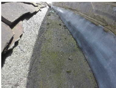
Cracked mortar to box gutter flashing Cement fillets to all edges and abutments are poor
