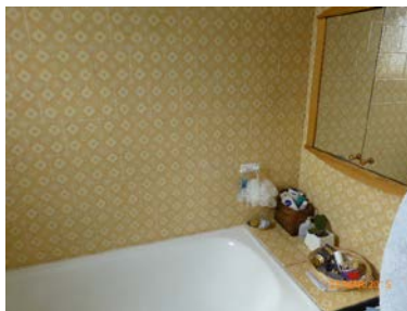
Wall tiling and sealant are in a poor state of repair
