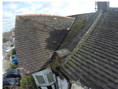
Pointing to the brickwork of the parapet walls is poor
