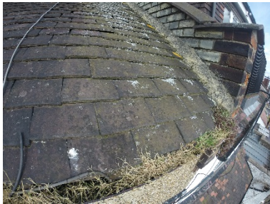
Gutters are blocked with leaves, moss and debris
