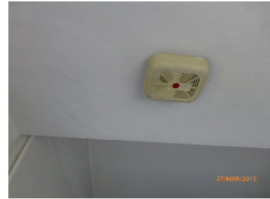
Battery powered smoke detection
