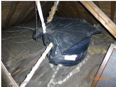
No bye-law 30 kits fitted to the water and expansion tanks
