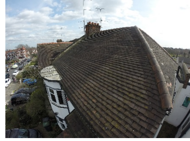
Front roof slope
