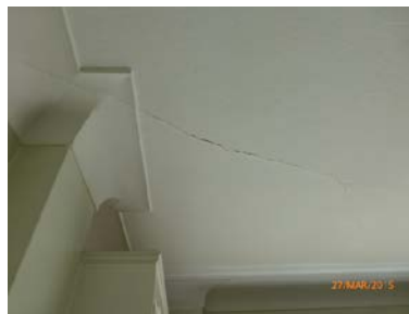
Cracks to the ceiling and coving
