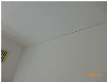
Cracks to the ceiling line
