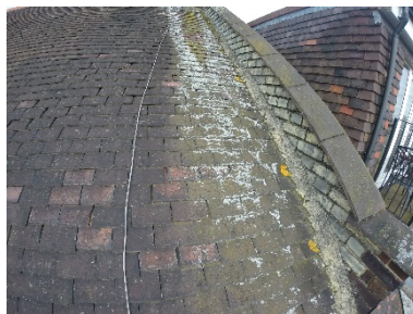
Cracked mortar to box gutter flashing Cement fillets to all edges and abutments are poor
