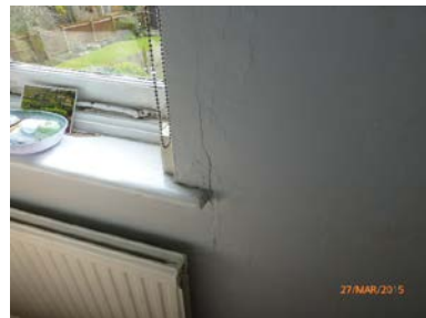
Cracks to the wall
