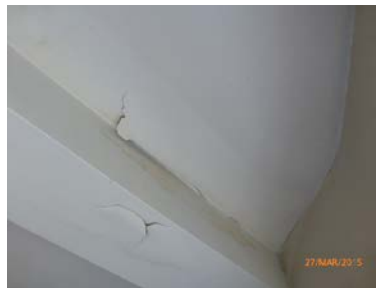
Water damage and staining to the drop down beam
