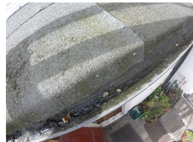
Rear shed roof is poorly felted and the flashing is poor
