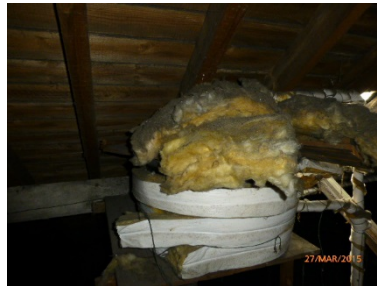
No bye-law 30 kits fitted to the water and expansion tanks
