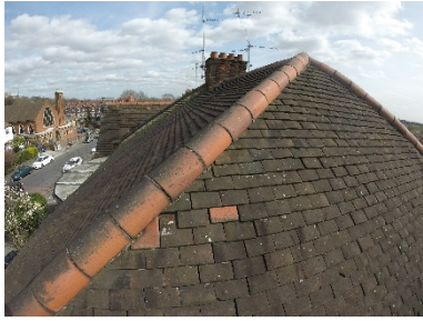
Damaged/missing/slipped tiles
