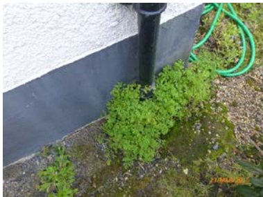
Leaking hopper
