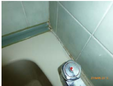
Sealant to the bath is poor
