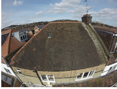
Rear roof slope
