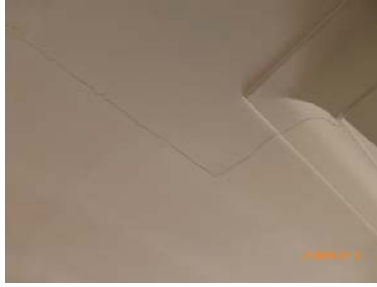
Cracks to the ceiling and coving
