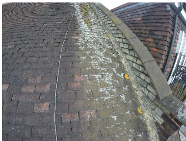
Pointing to the brickwork of the parapet walls is poor
