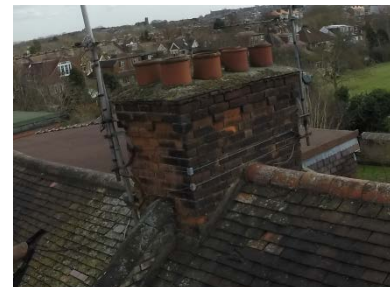
Open chimney flues
