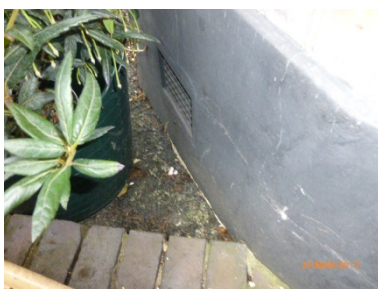
Small air bricks in the front wall
