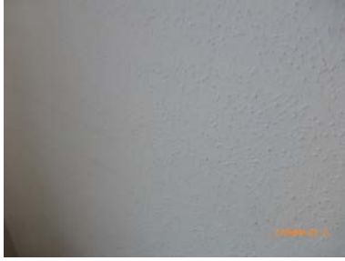
Wall have a textured coating
