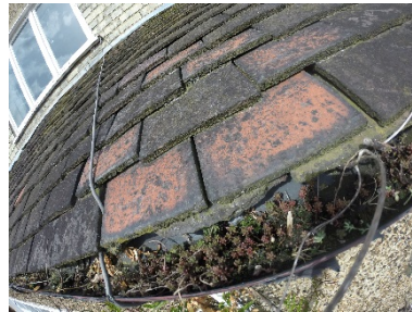
Gutters are blocked with leaves, moss and debris
