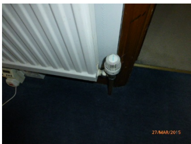
Thermostatic radiator valves
