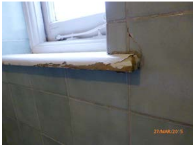
Sill in shower is water damaged
