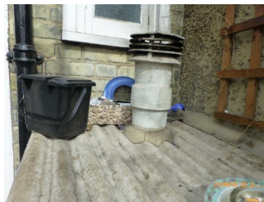
Flue through the roof
