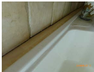
Sealant to the worktops is poor
