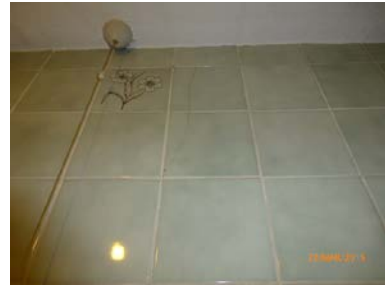
Crack to the wall tiles
